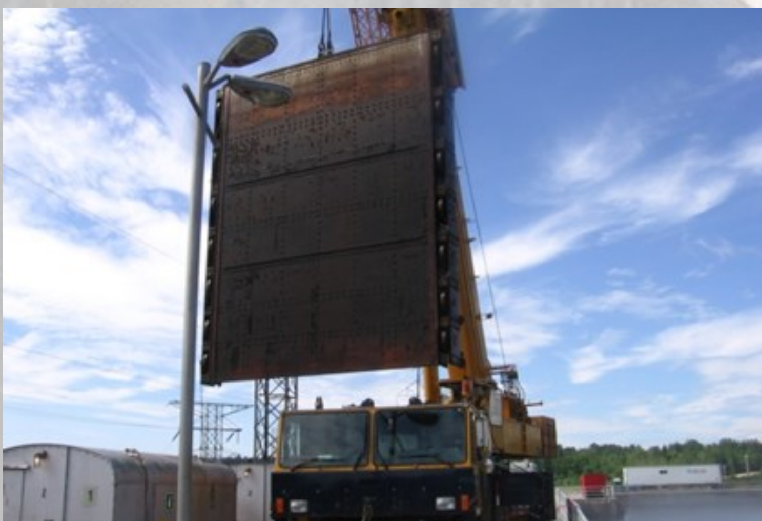
Old Intake Gate
