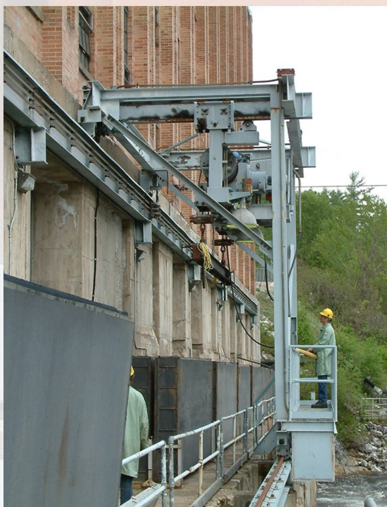
Downstream Gantry Crane Before
