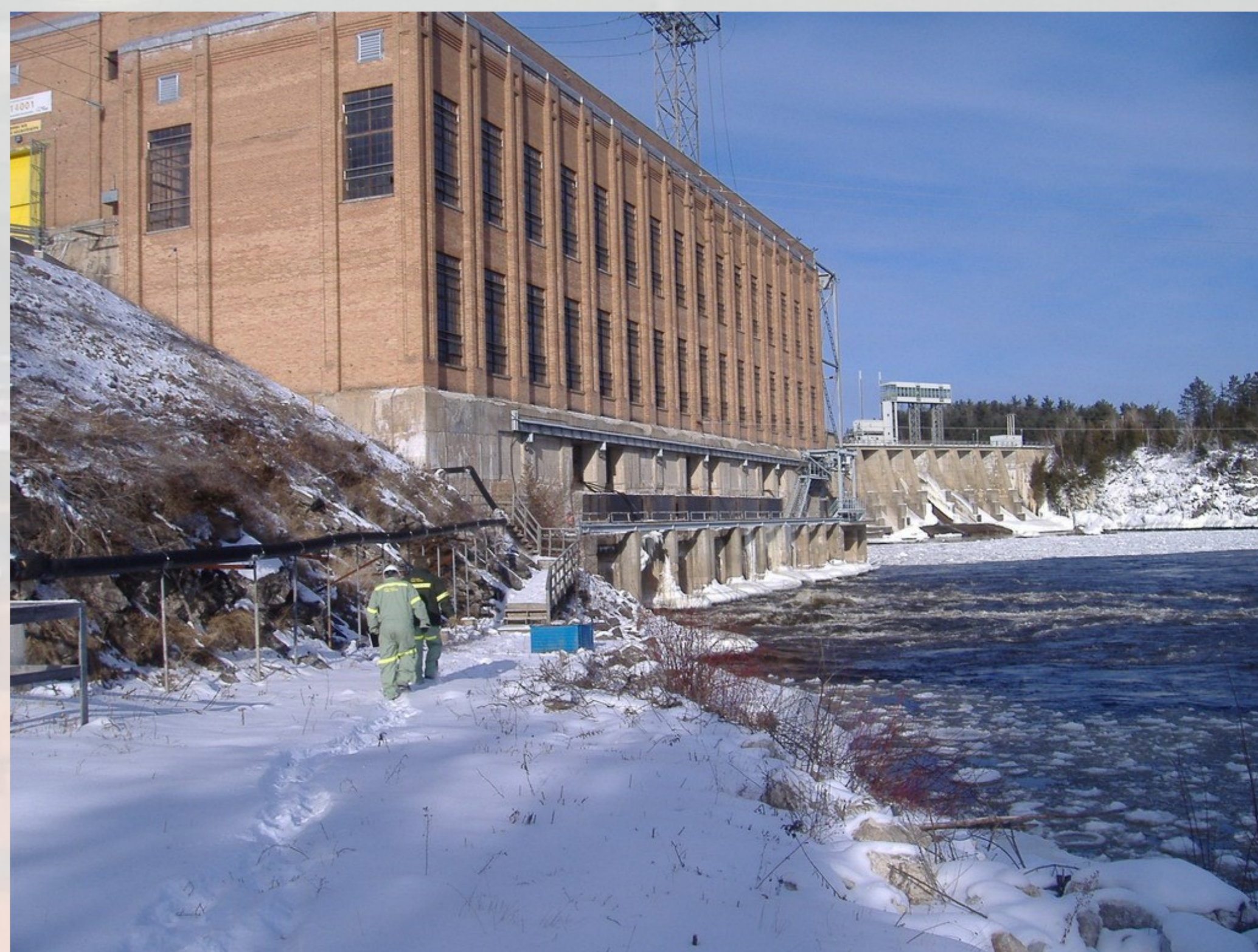
Downstream View - Powerhouse
