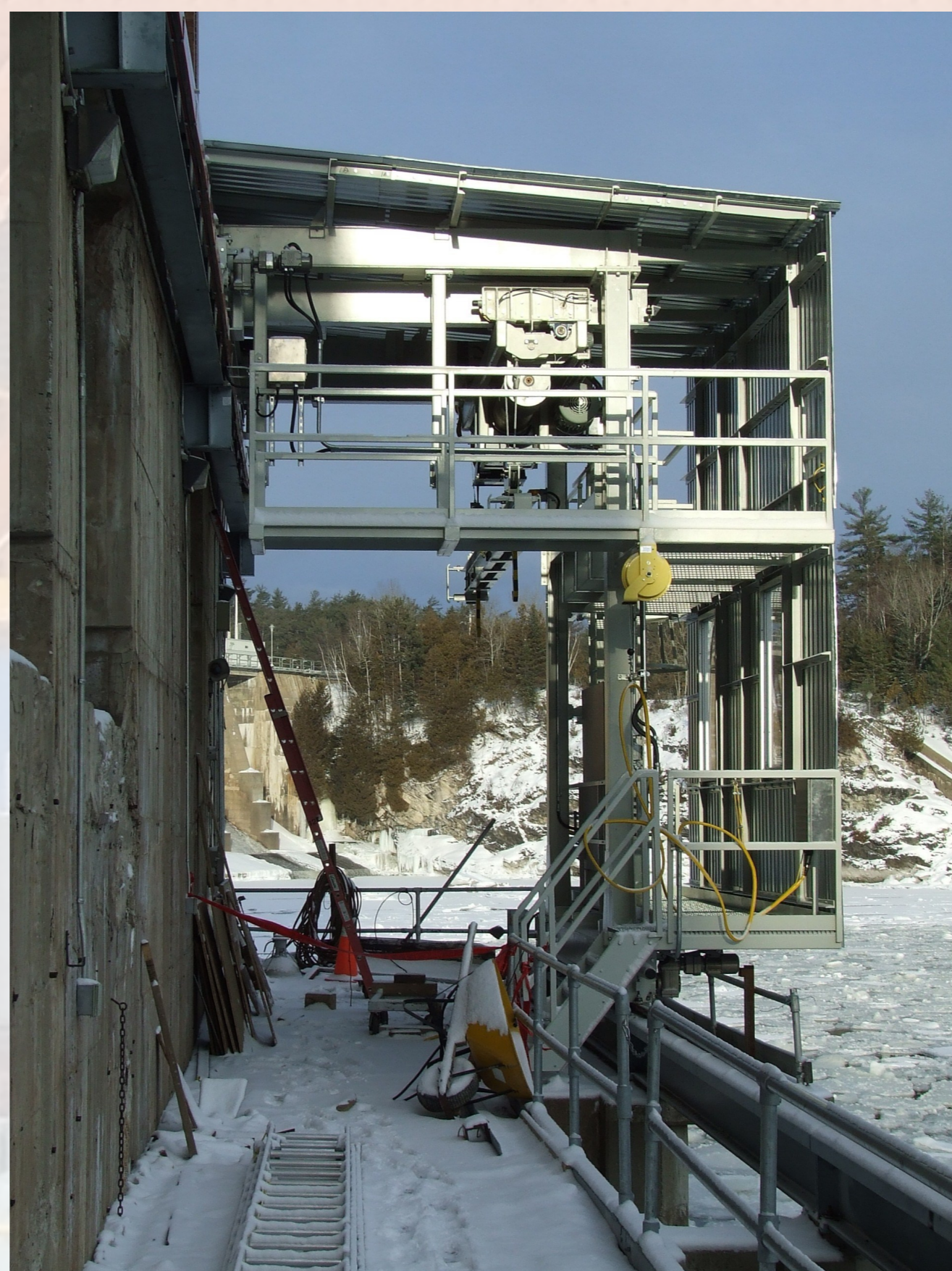
Downstream Gantry Crane After
